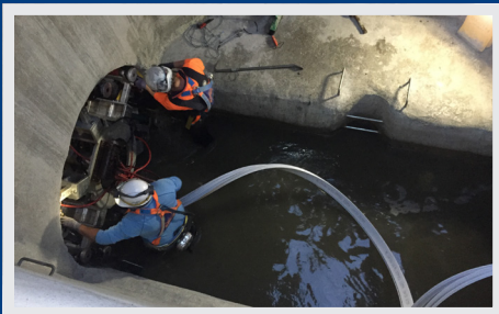
Setting up the Rotaloc winding machine
