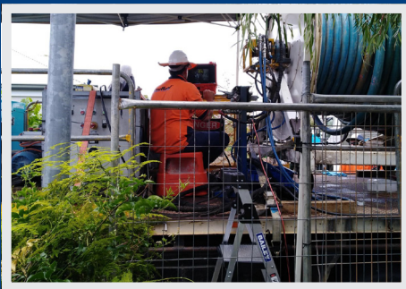
Rotaloc machine operator lining the pipe by remotely controlling the machine.
